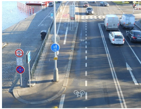
Fig. 13 Nábřeží Ludvíka Svobody street (parallel usage of bicycle lane and bicycle path); source: Authors.
