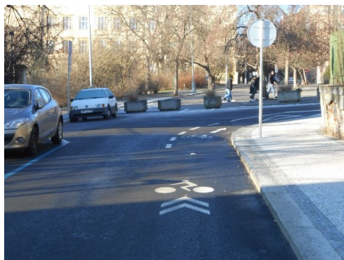
Fig. 11 Hradešínská street (potential danger due to the sharp curve of the street); source: Authors.
